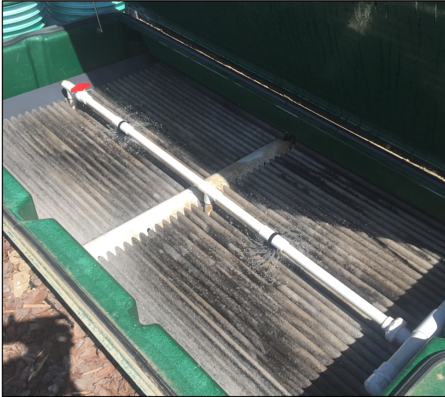
Spinner Nozzles Check spray coverage
